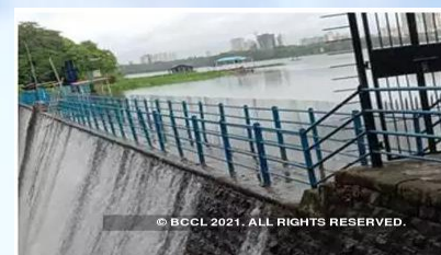
Powai lake overflows
